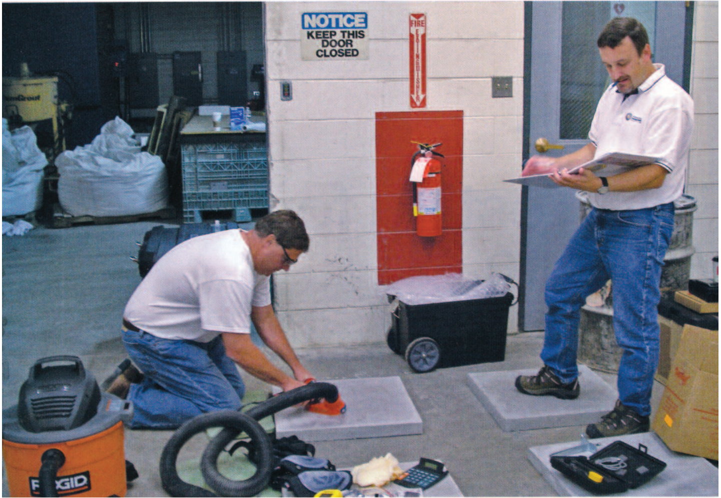
The in situ relative humidity test also needs to be conducted properly to provide consistent and meaningful results.
